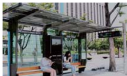
<PV on bus stations>
